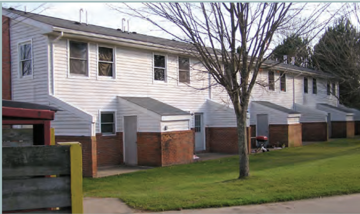
Rear view of the Washington Square apartments, showing the current layout of the concrete pads behind the units.
