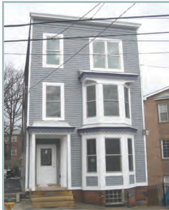
58 Crawford Street, after rehab
