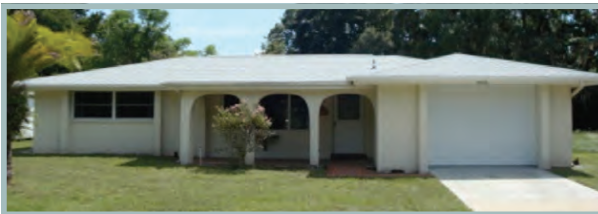
Before and after photos of house renovated by Tampa Bay CDC and Pasco County Community Development Corporation with NSP funds.
