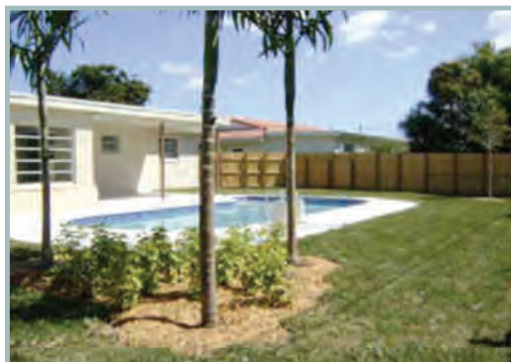
Before and after photos of a house acquired and renovated with NSP assistance in Broward County.
