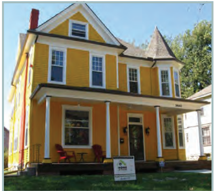
Bish's house fully remodeled and ready for occupancy.
