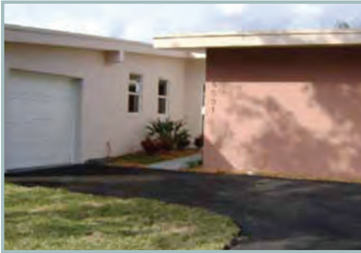
A home newly renovated with NSP assistance.
