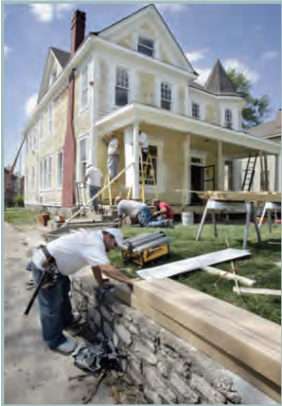
Bish's house during the renovation process.
