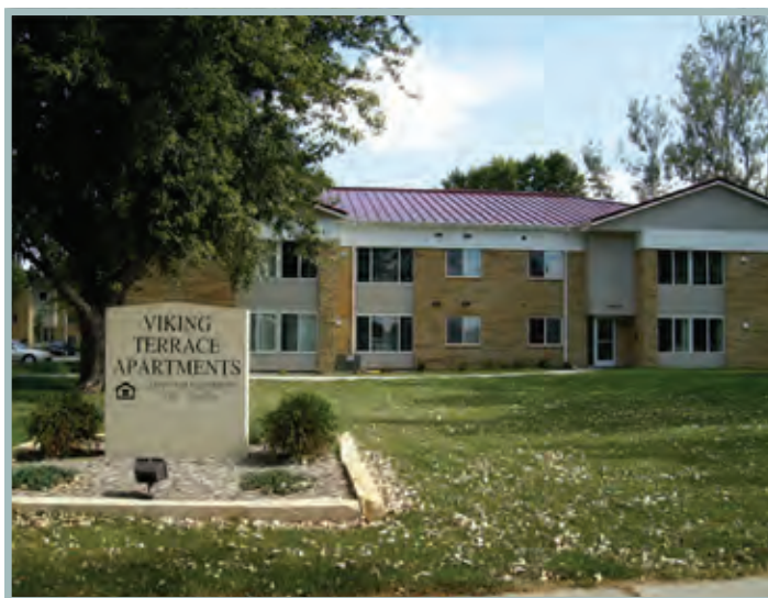
The Viking Terrace Apartments after renovation. SWMHP improvements included new roofs and siding.
