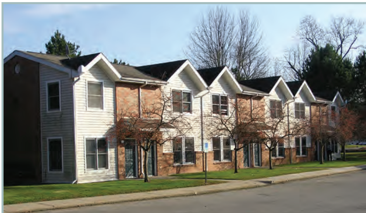
Washington Square Apartments in Barberton, OH, a joint partnership between NDS, the city of Barberton, Summit County, the Ohio Housing Finance Agency and the Akron Metropolitan Housing Authority.
