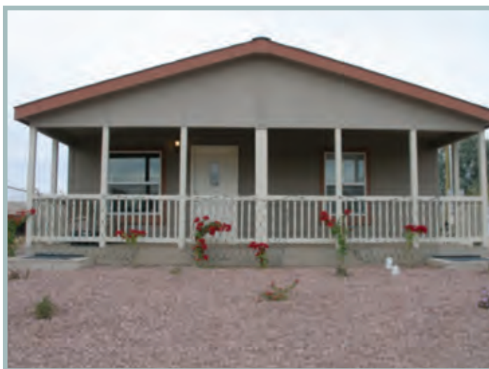
Primavera replaced this deteriorated house on West 38th Street with a new, attractive energy-efficient unit.
