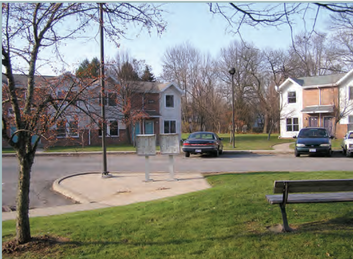
View of the exterior at Washington Square. While the buildings look well kept, it was the interior of the units that posed the rental challenges: small three-bedroom units, no air conditioning, poor insulation and electric heat.
