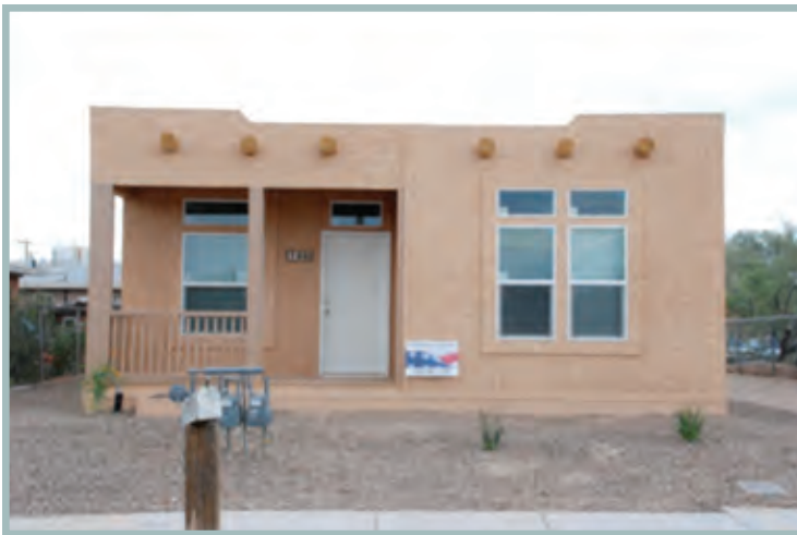
Before and after photos of house on West 27th Street. Primavera demolished and replaced using NSP1 funds.
