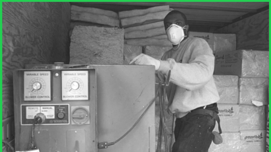
Insulation Installer with Blower Machine and Various Insulation Types
