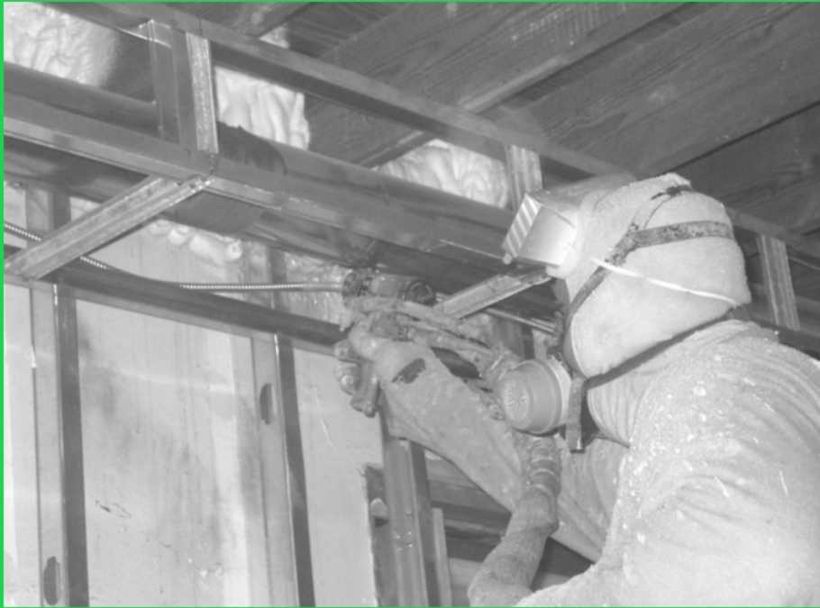
Spray-foam Insulation
